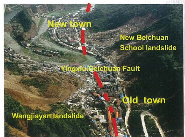
Figure 4. Beichuan county town seat (looking northeast). The Yingxiu-Beichuan fault runs right through the old county town. Post-earthquake Wangjiayan landslide (front) and new Beichuan high school rockfall (back) are shown.
