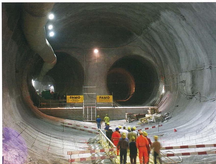
Figure 3. Tunnel branch-off structure with 320 m 2 cross section
