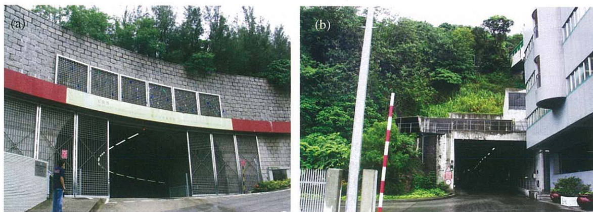
Figure 3. Cavern portals of (a) Stanley Sewage Treatment Works and (b) Island West Refuse Transfer Station
